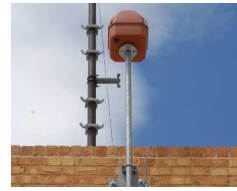
(c) Installed antenna node
